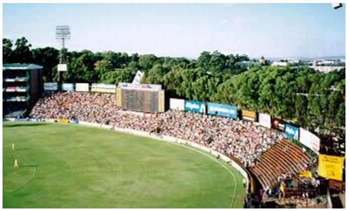
Fig : New Wanderers Stadium, Johannesburg.
